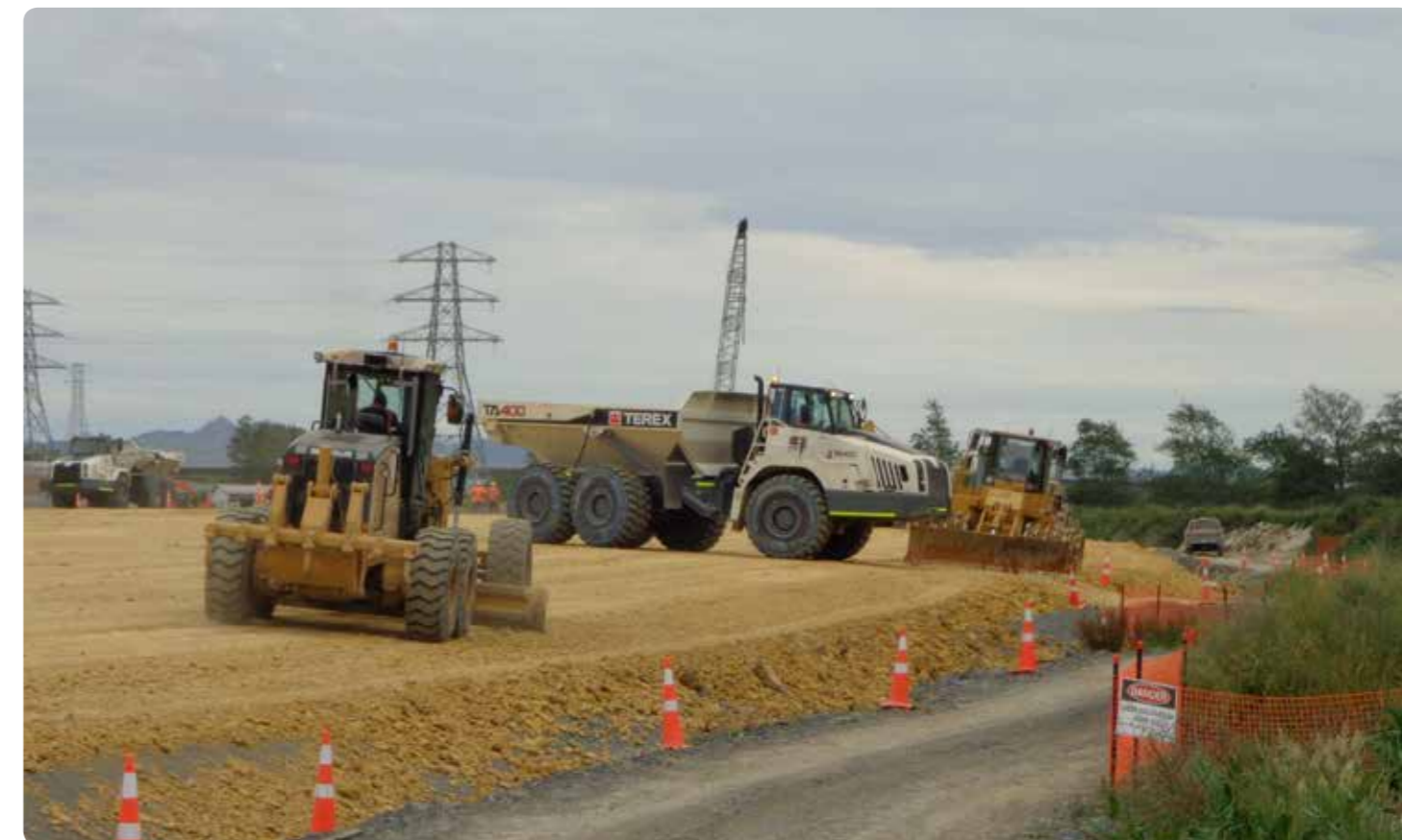
Moving ahead: Bulk fill earthworks have been under way lately
