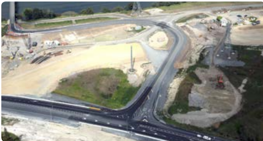
The temporary road at Rangiriri servicing the Glen Murray bridge
