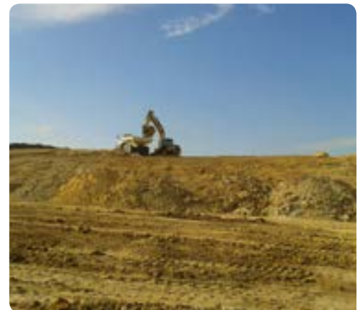
Earthworks: About 75,000 cubic metres of earth is being moved a month
