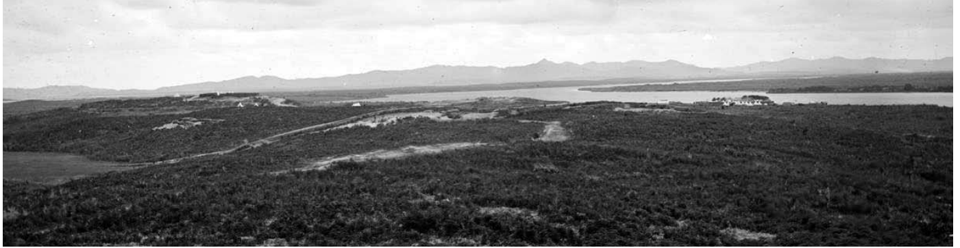
Photographs by Beere taken soon after the battle in 1863. It shows the main line of Maaori fortifications across the Great South Road with the newly constructed British redoubt in the background.
