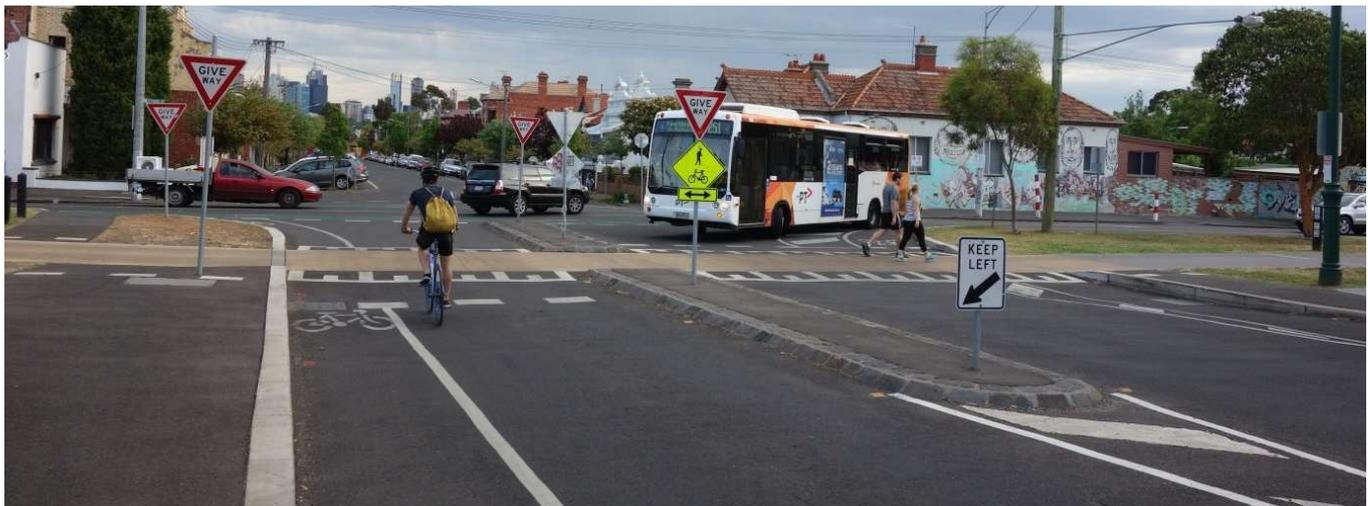
**Figure 9: Bent-out crossing on busy bus route with offset too short for buses (photo: Axel Wilke)**
