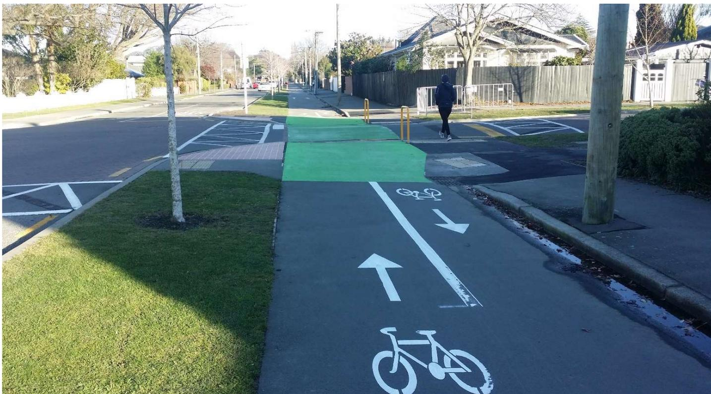
**Figure 7: Straight layout with minimal offset**
