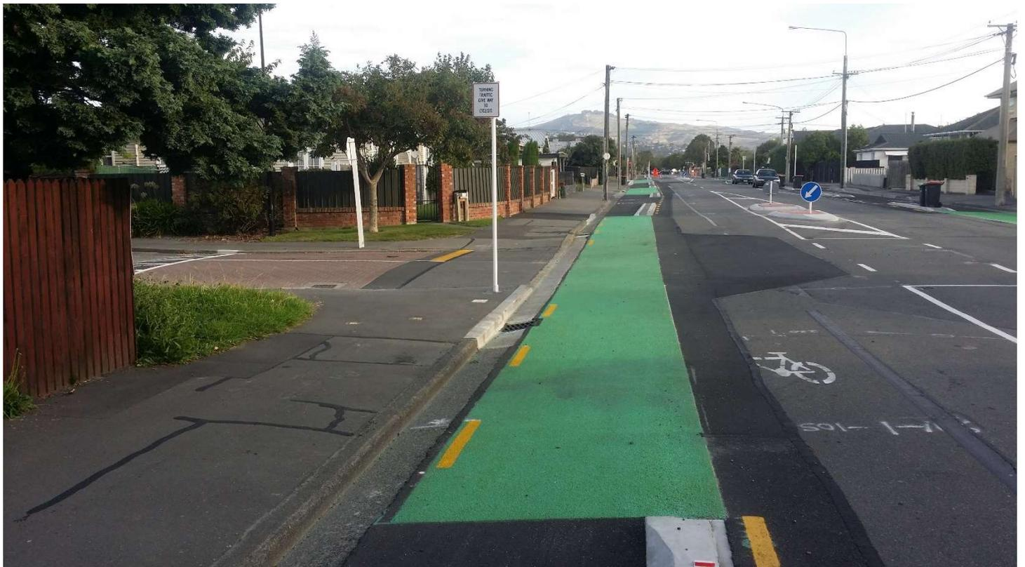
**Figure 6: Straight through cycleway, Antigua Street Christchurch (separator stops short of intersection)**
