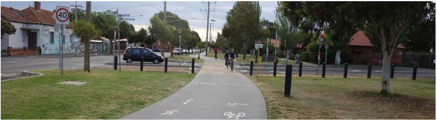
**Figure 10: View of offset that is insufficient for bus drivers on busy bus route (photo: Axel Wilke)**
