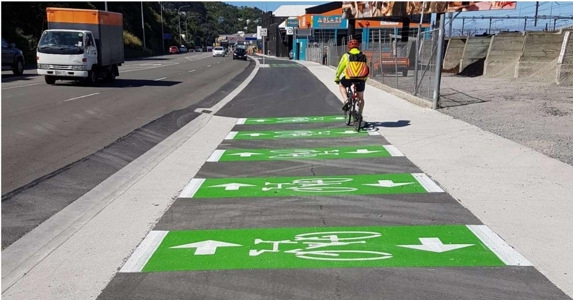
**Figure 15: Separated bi-directional cycleway with adjacent parking at a commercial driveway**
