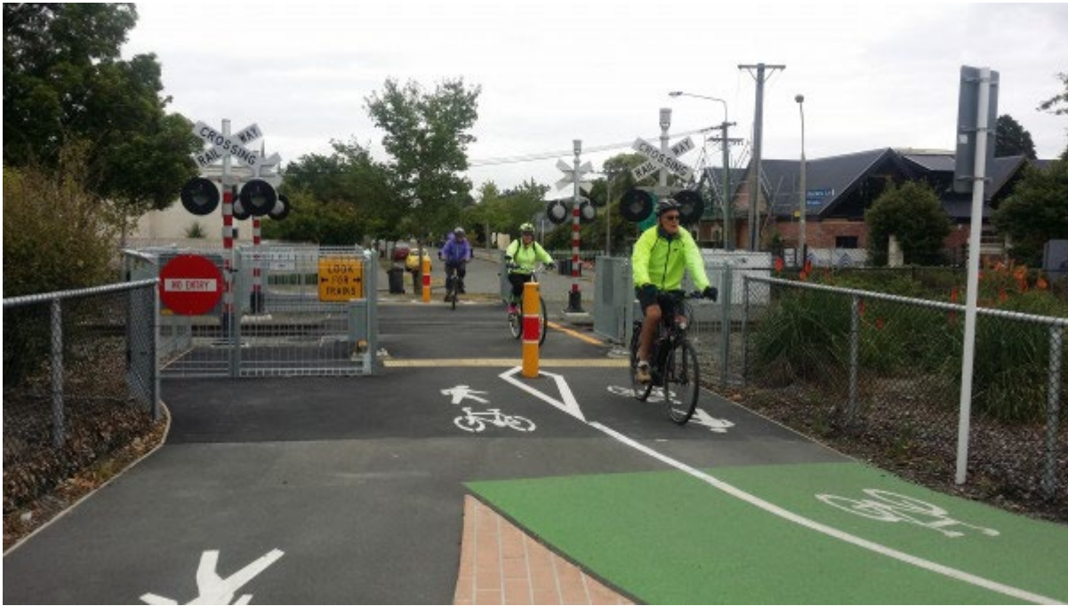
Figure 42: Shared path and automatic pedestrian gates at Matai Street, Christchurch. (Photo: Glen Koorey)
