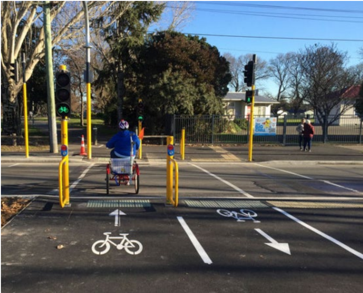
Figure 33: Pedestrian and cycle crossing with separate signals, Linwood Avenue in Christchurch. (Photo: John Lieswyn)
