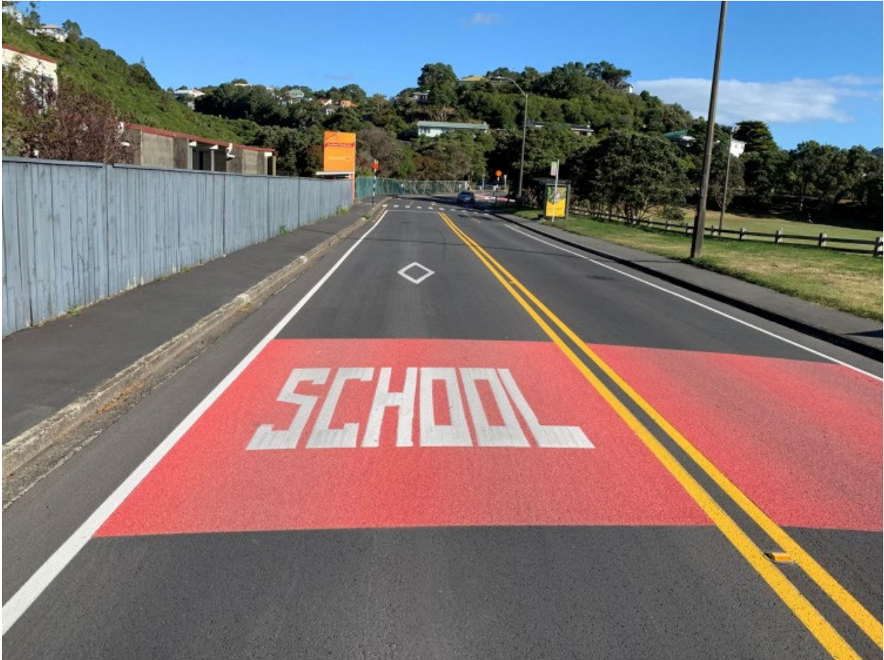
Figure 39: SCHOOL marking on red block prior to zebra crossing. (Photo: Simon Kennett)
