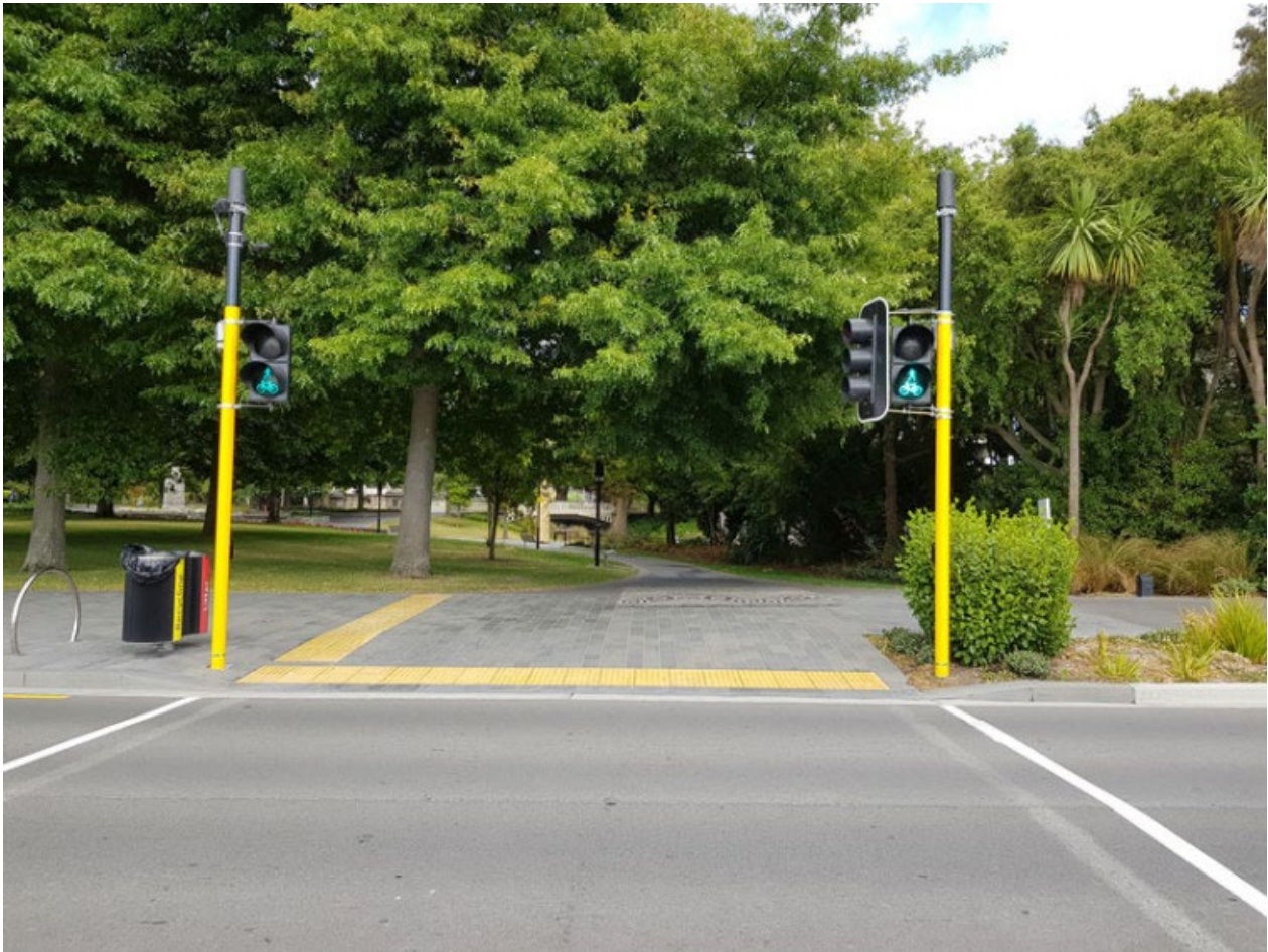
Figure 34: Combined pedestrian and cycle signal display (Photo: Gemma Dioni)
