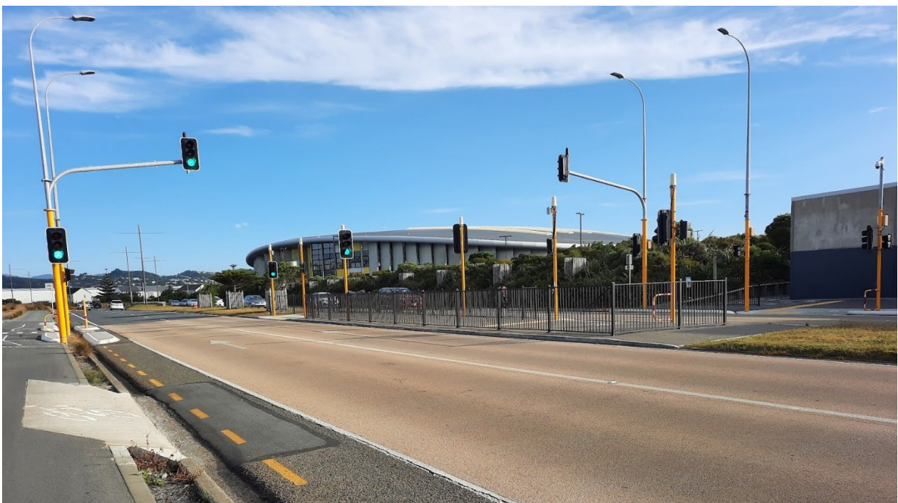
Figure 30: Two-stage crossing for pedestrians. (Photo: Lorelei Schmitt)
