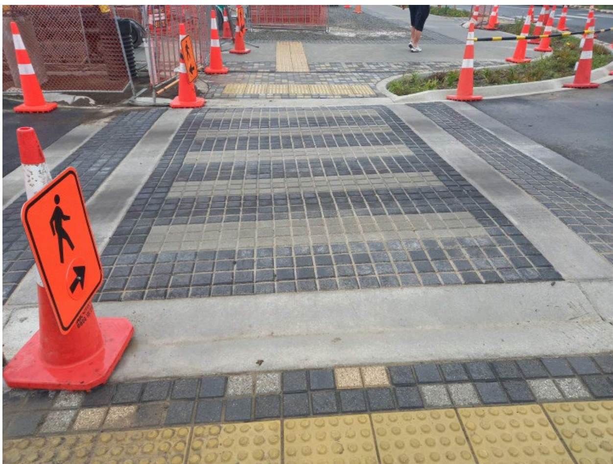
Figure 24: Paved zebra crossing providing insufficient contrast of white bars. (Photo: Jeanette Ward)
