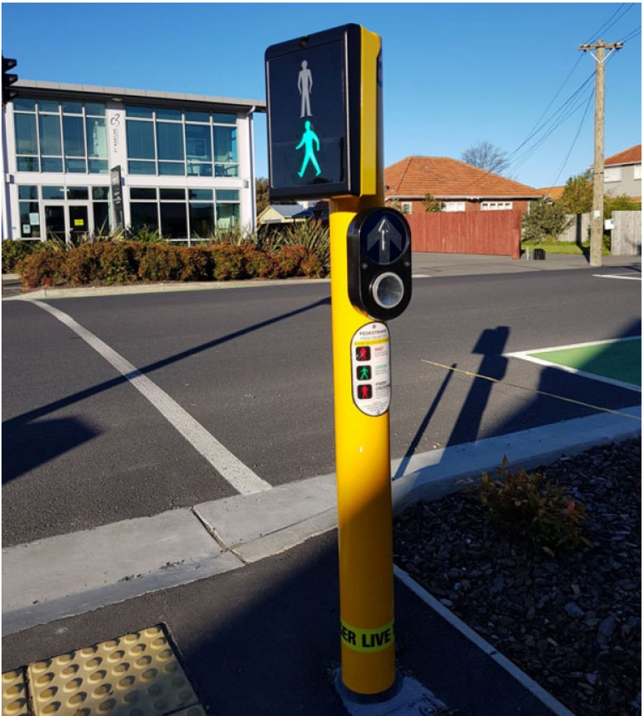
Figure 32: Nearside pedestrian signal display. (Photo: Gemma Dioni)
