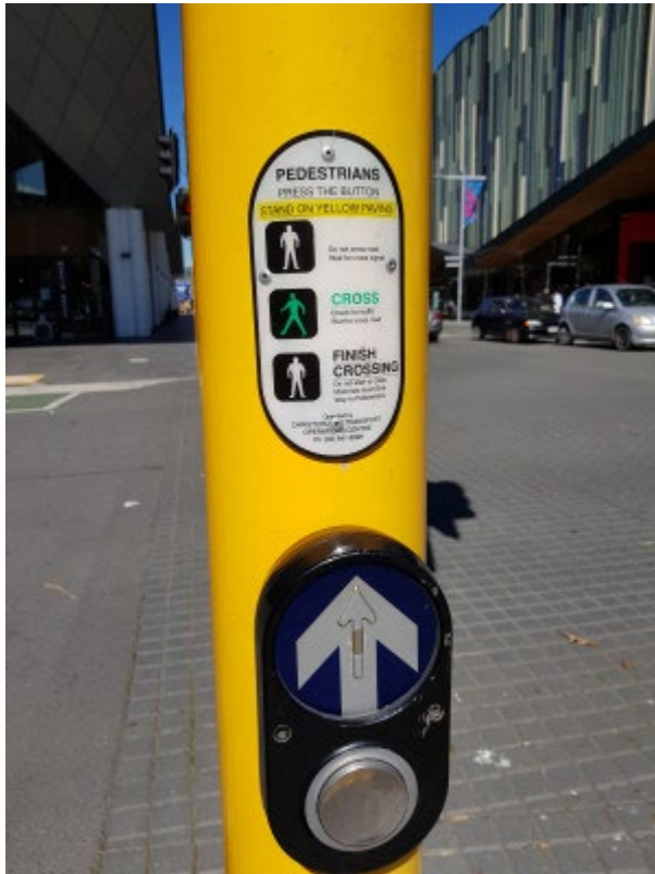
Figure 35: Pedestrian push button with explanatory placard. (Photo: Gemma Dioni)
