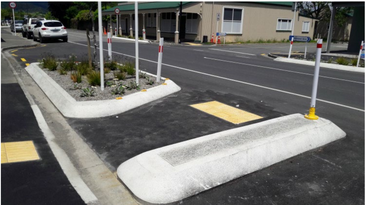
Figure 12: Retrofit kerb extension, Brightwater. (Photo: Jeanette Ward)
