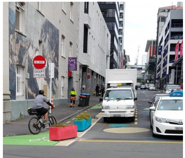
A traffic filter can help establish a contra-flow cycle lane, as pictured here on Federal Street in Auckland.
