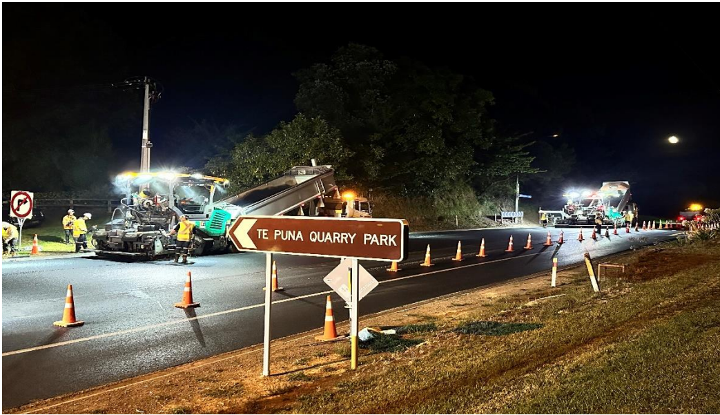
Photo: SH2 Snodgrass Road rebuild
