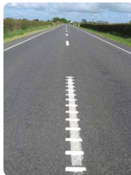
Rumble strips may be laid along road edgelines (left) or centrelines (right)
