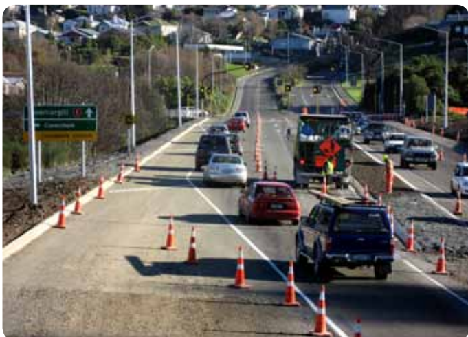
The new highway layout looking south toward Barnes Drive
