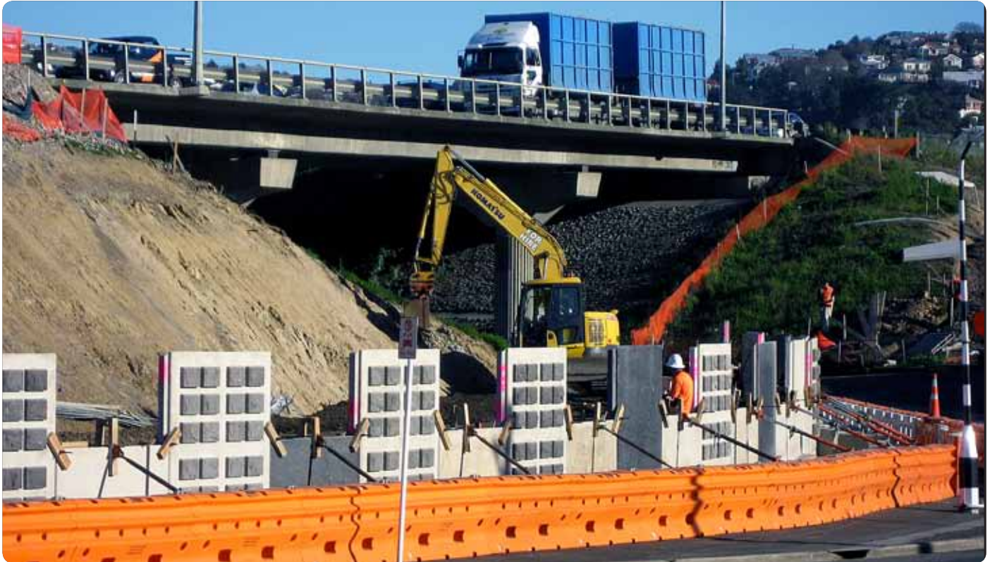
Retaining walls being installed on Bridge Street
