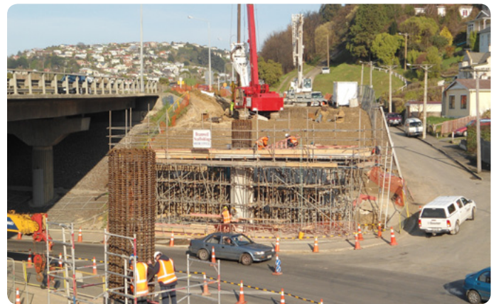
Glen Bridge construction
