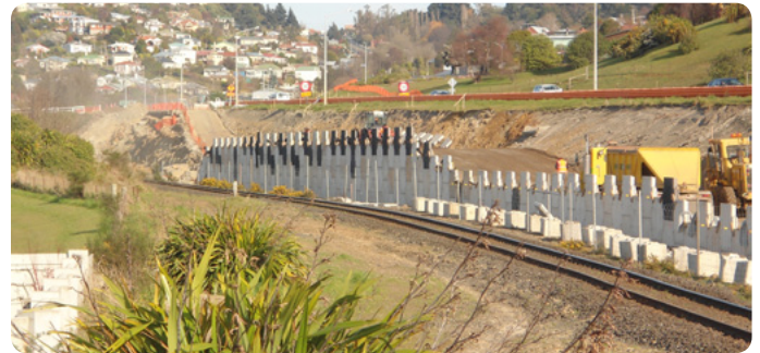
Retaining wall construction
