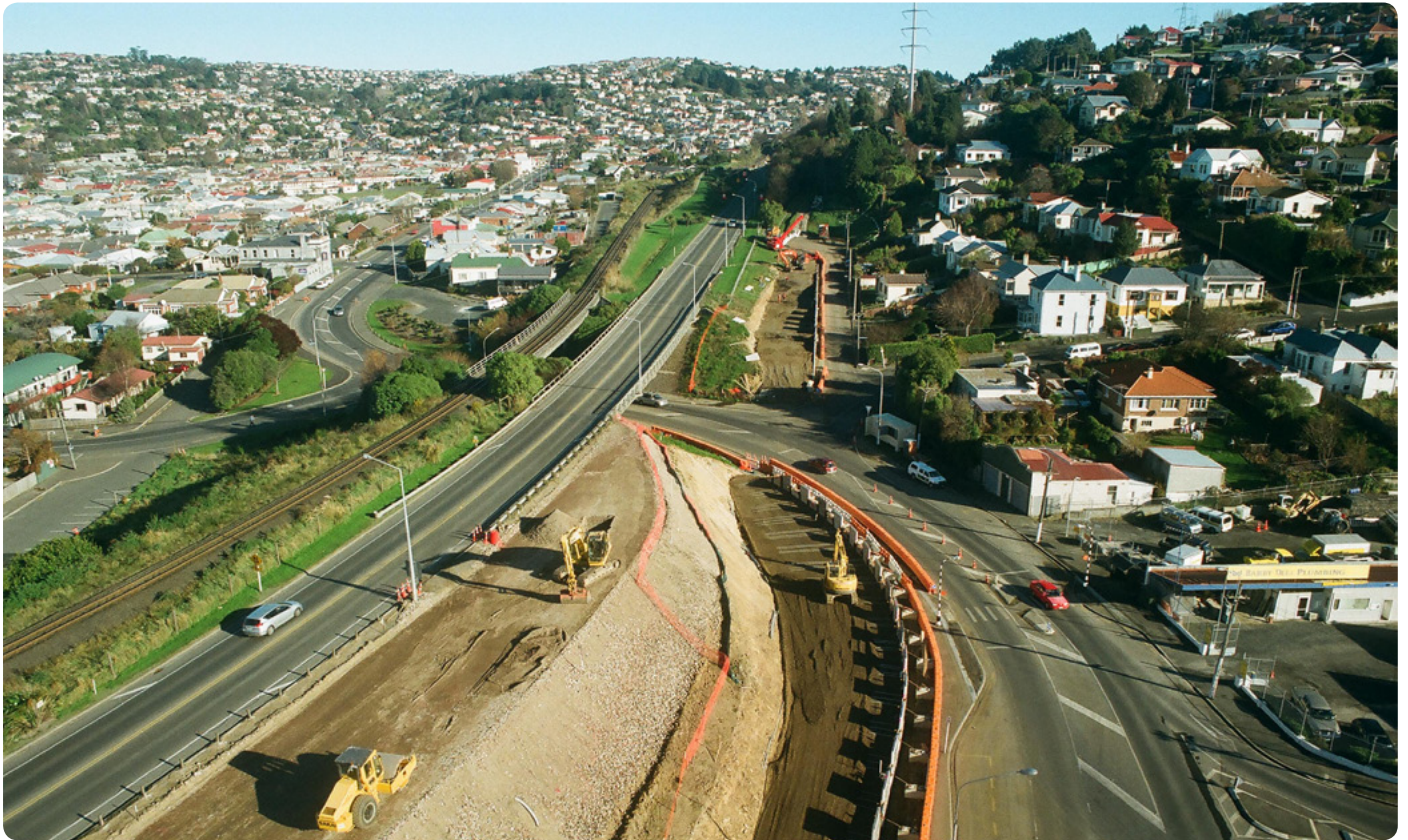
Construction work in the Glen Bridge area looking south
