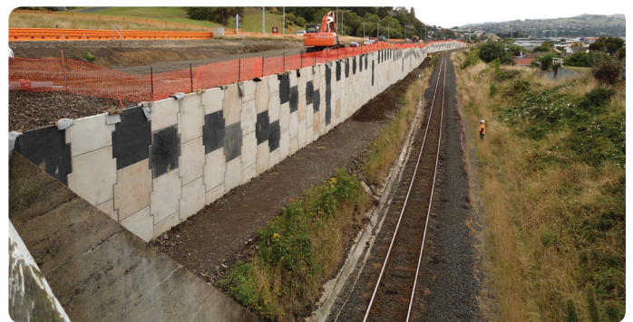
The retaining wall alongside the main trunk railway nears completion
