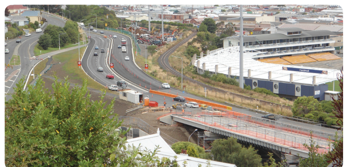
Decking on the new Glen Bridge overbridge
