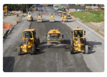
Once all zones are completed to this point we need to let traffic run on the chipseal surface for a period of time to allow for minor settlement. Then final surfacing (asphalt) will be laid.
