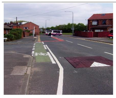
Speed cushions are small rectangular humps, resembling a seat cushion in shape. They are approximately the width of a car and usually placed in rows of 2 or 3 across the road width. Cushions are rarely used individually but tend to form a series on a street or across as an area-wide treatment to maintain uniform speeds. Cushions are particularly good at offering traffic calming benefits without significant adverse effects on bus or emergency service access.
