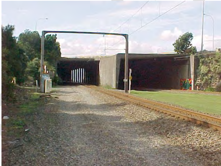
Figure 8-8 - Southern Rail Overbridge Cells
