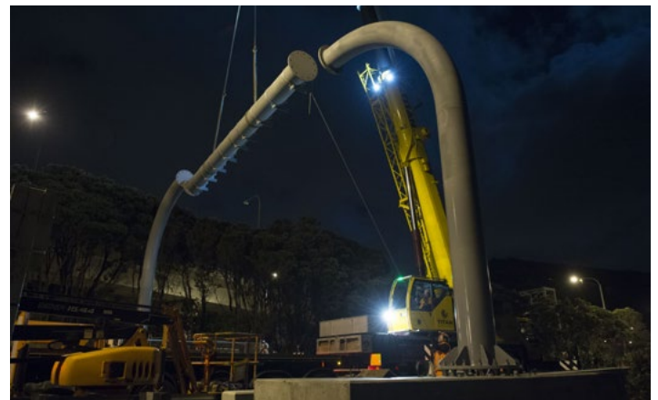
Lifting the beam of the SH2 off-ramp portal gantry.
