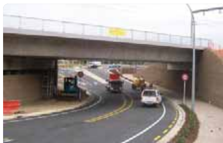
NORTON RAIL BRIDGE. The new Norton Road connection to the Rifle Range Road Roundabout was opened to traffic on 27 September 2008
