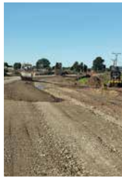
Railway line earthworks
