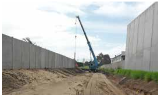
Installing the 70 concrete panels along the new railway corridor
