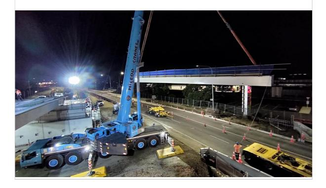
Achieving this milestone also finishes beam installation on all three of Bay Link's bridges. Beam installation began in February 2021 with the first bridge, which spans the East Coast Main Trunk railway line, and continued in July 2021 on the second State Highway 2 (SH2) bridge. Both of these bridges are now open to road users as part of the SH2/29A Te Maunga interchange.
