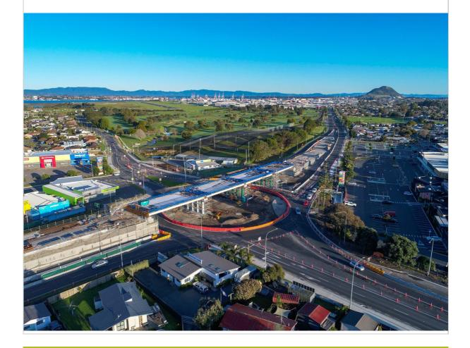
In total, 46 bridge beams, all locally manufactured in Te Puke, have been placed. Installation has predominantly been completed at night when traffic flows are lowest and the airspace is available for cranes, which, at times, have extended almost 65 metres above sea level, to lift the large reinforced concrete beams into place with precision.
