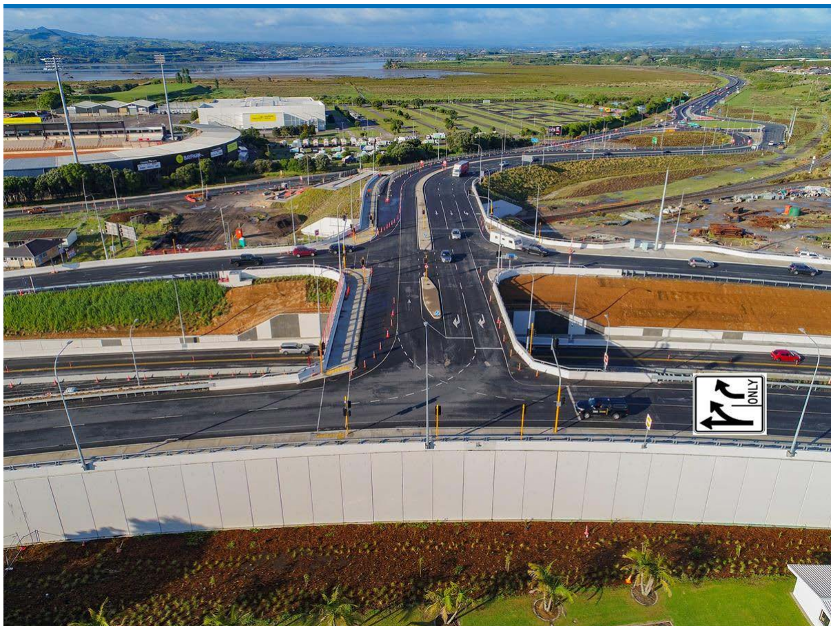
New lane configuration at SH2/SH29A Te Maunga interchange
