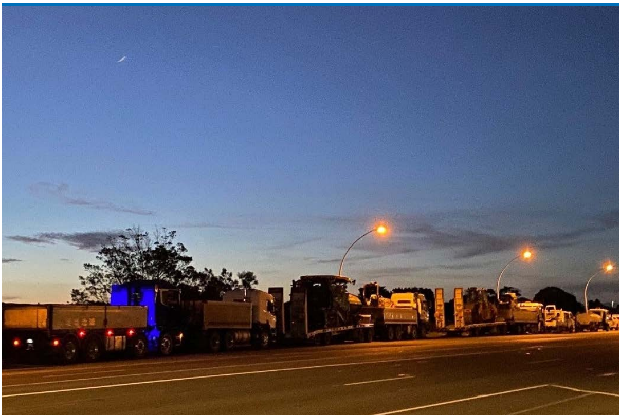
Crews preparing for nightworks
