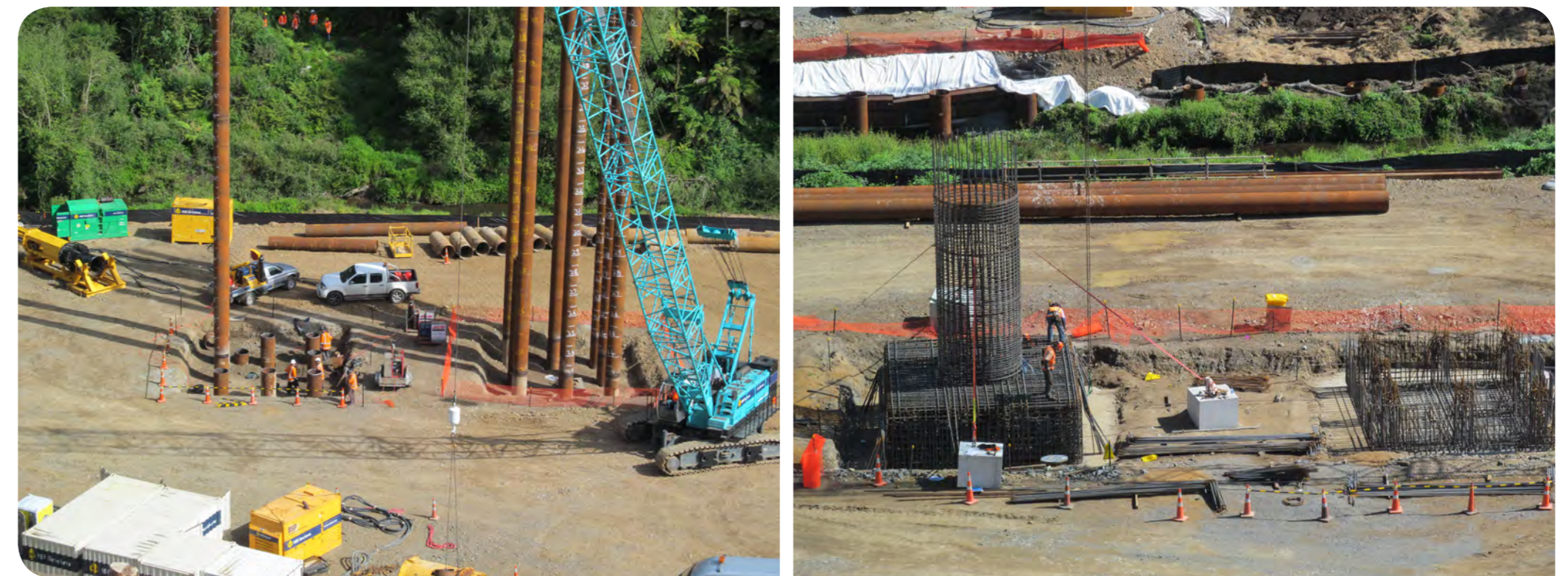
The piles are made from 711mm diameter casing driven into the ground and filled with concrete. The casing is 16mm thick and an 80mm thick driving plate is welded to the driving end of the pile.
