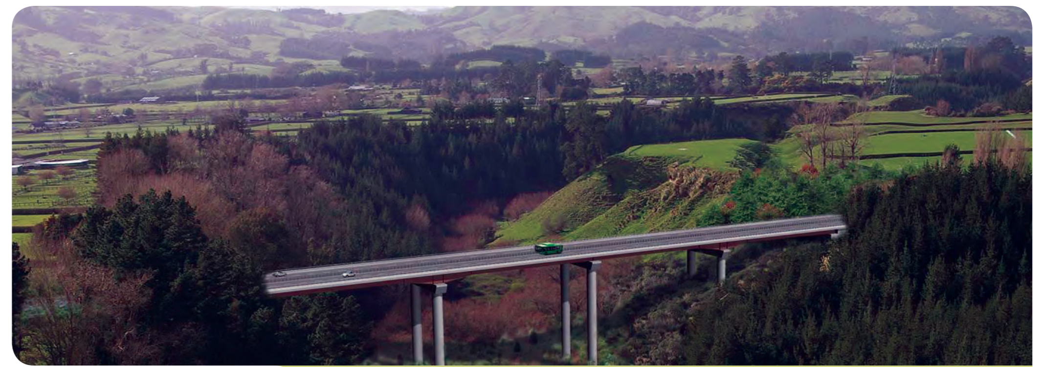
Artists impression of the completed Karapiro Gully Viaduct.
