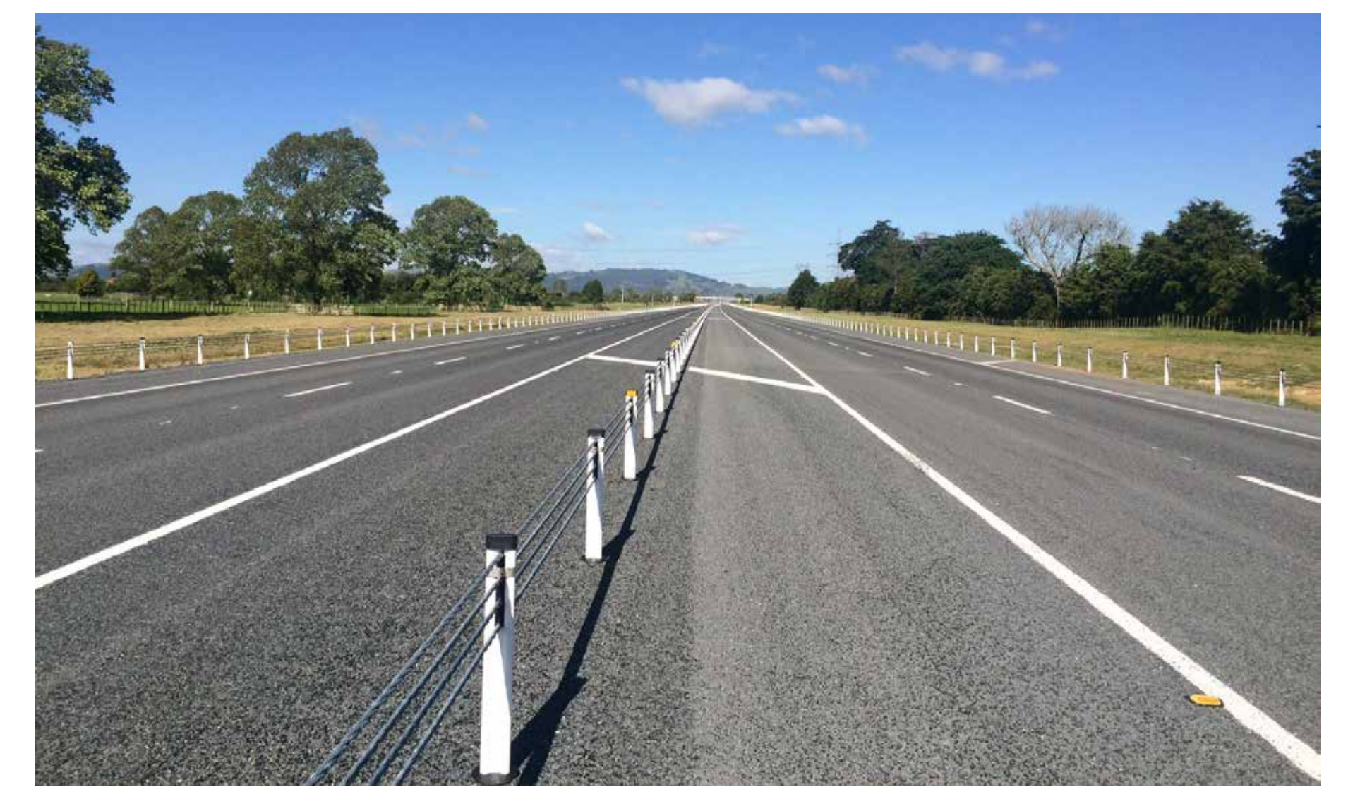
There is approx 192km of wire rope used in barriers and approx. 30,300 litres of paint was used for pavement marking
