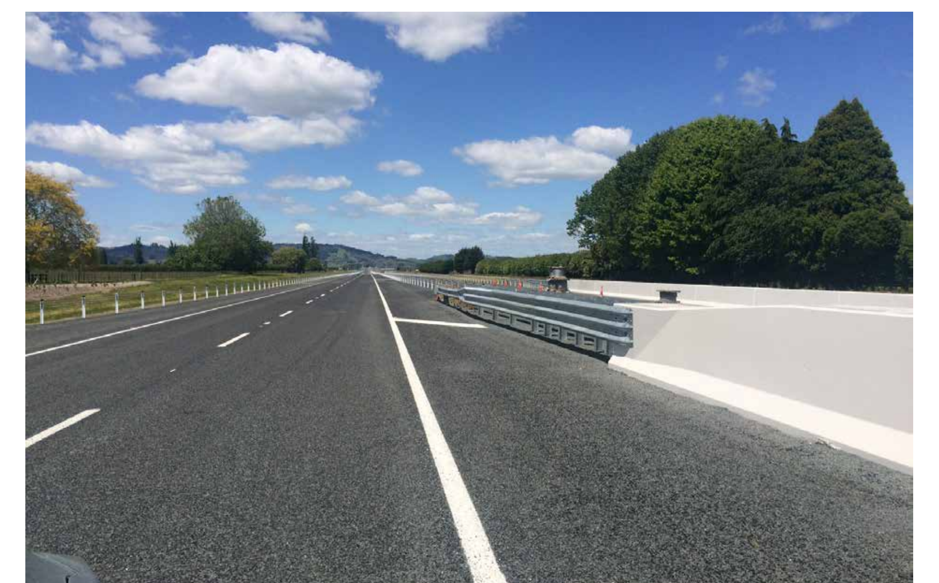
Approx. 2km of concrete crash barriers and 4000 traffic cones were used on site
