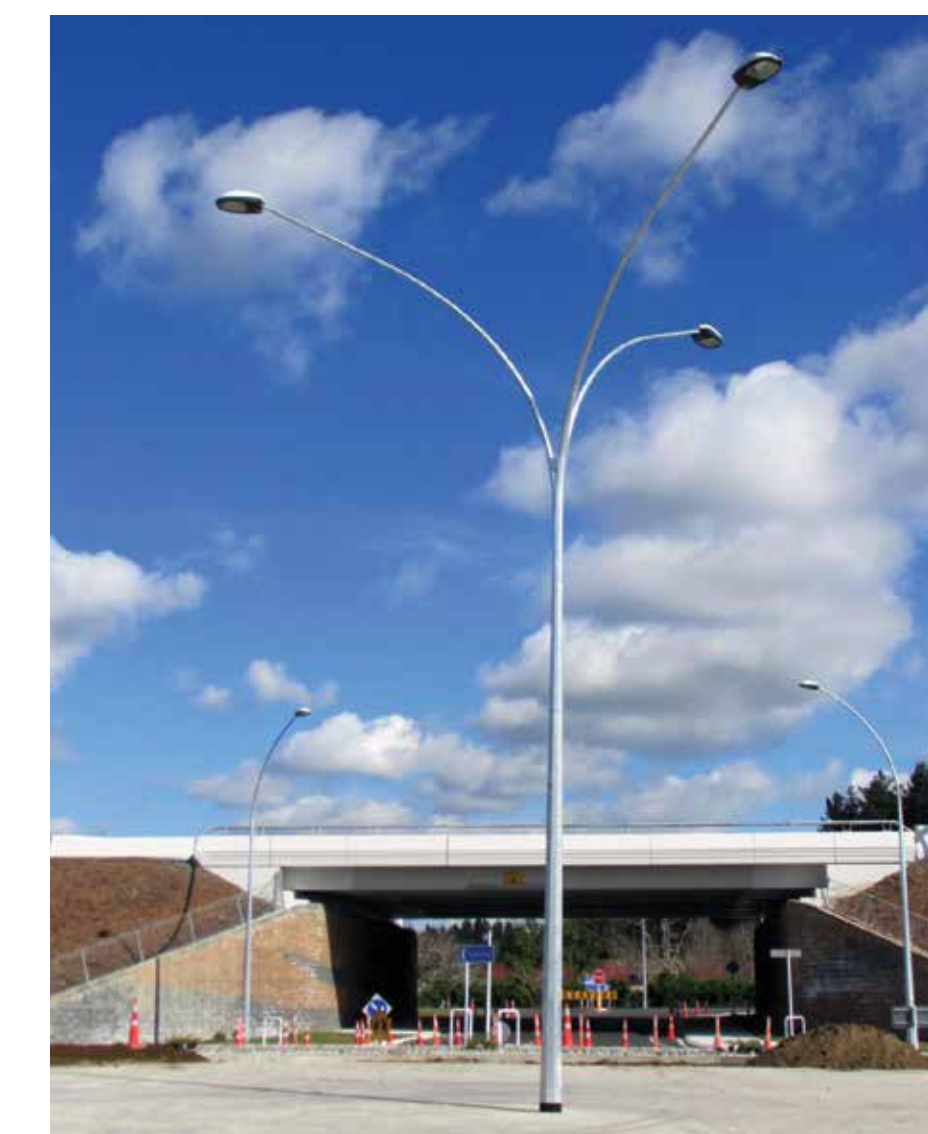
The voltage of the street lighting is only 230 volts, similar to a wall socket in your home
