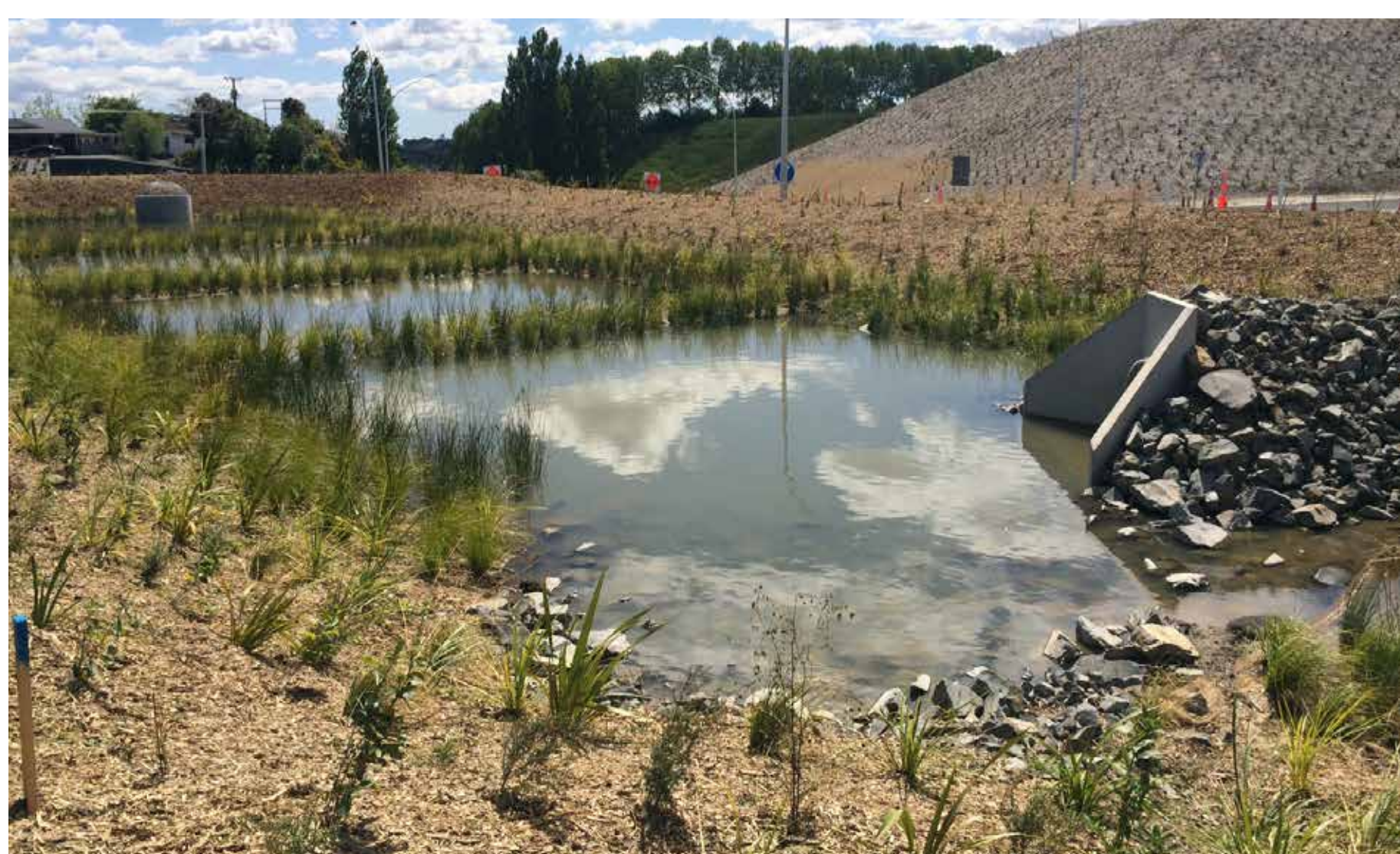
Newly planted native grasses around a stormwater pond
