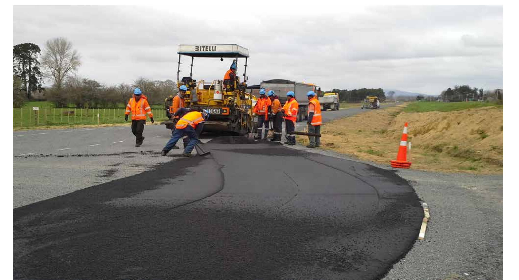
OGPA being laid
