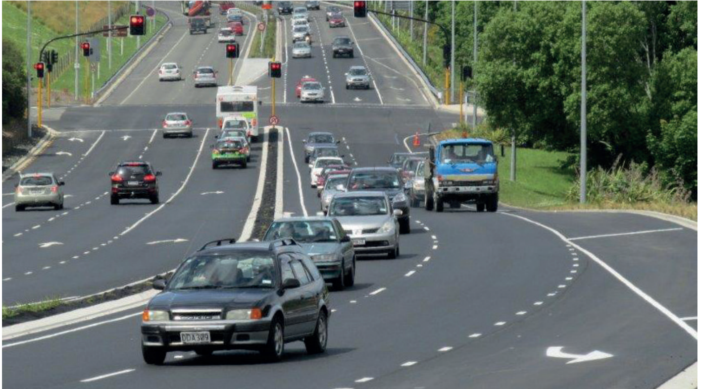
An upgraded section of SH1 Caversham Valley near Barnes Drive
