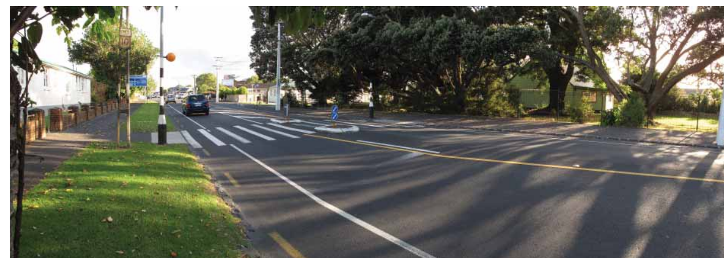
Figure C-6.13: Photo 6-3 Carrington Road, where the cycleway links from Sutherland Road
