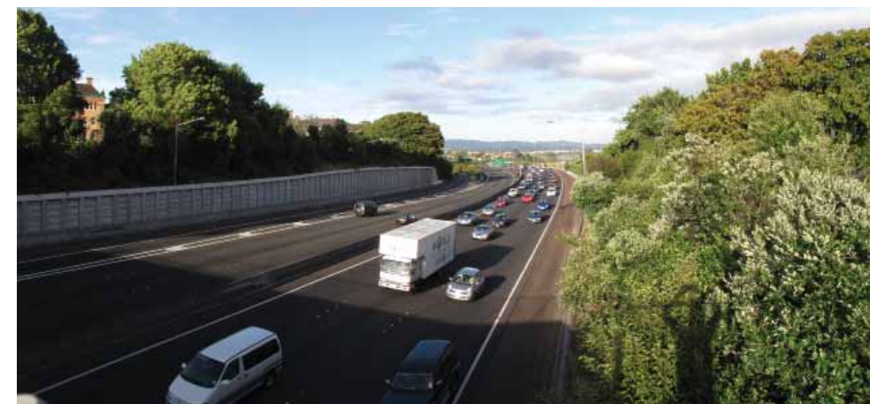
Figure C-6.11: Photo 6-1 View west along SH16
