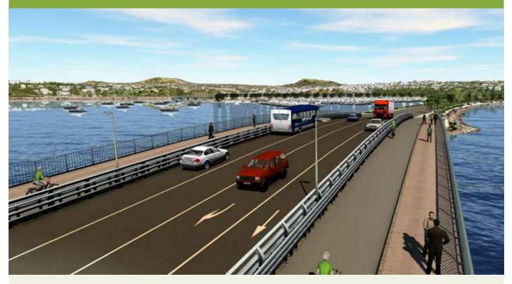
Better walking and cycling amenities on Ngapipi Bridge are a key part of the wider programme of improvements in the area. We propose installing 2.5m-wide 'clip ons' on both sides of Ngapipi Bridge to provide new footpaths and converting the existing footpaths into cycleways. The existing footpath on the northern (seaward) side of the bridge will become a separated two-way cycleway, while the shared path on the southern side will be converted into a one-way, on-road cycling route.
