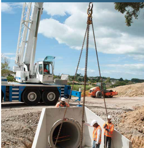
A large 1.5 metre culvert channels water underneath the path.
