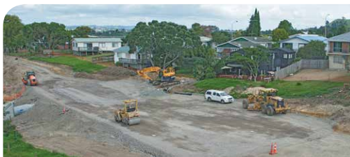
Building up an earth ramp to create a gentler slope.
