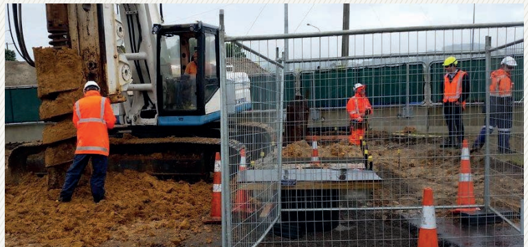
Auger drilling at Maungatapu roundabout
