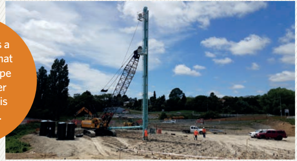
Installing wick drains near Hammond Street
