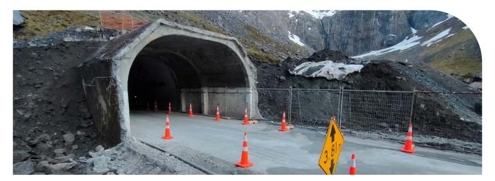
A steady stream of the approximately 150 pre-cast concrete modules required for the new shelter are regularly arriving on site. The wall on the southern side of the shelter is clearly visible as you can see in the photo below. These modules are made off-site then transported to the tunnel for assembly.
