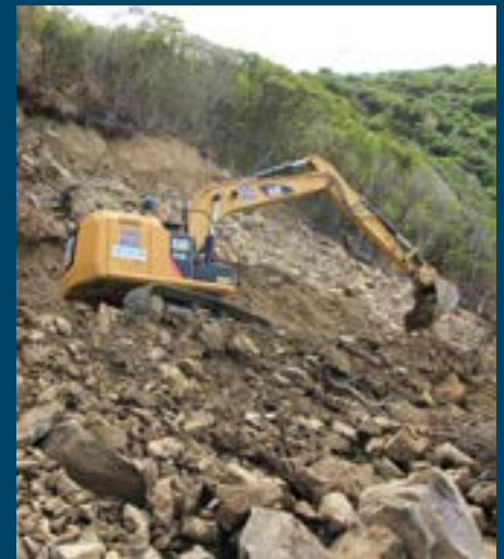
Ford Brothers excavator clearing a secondary slip around Site 2
