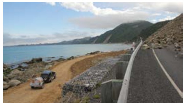
The construction access track around Site 2
