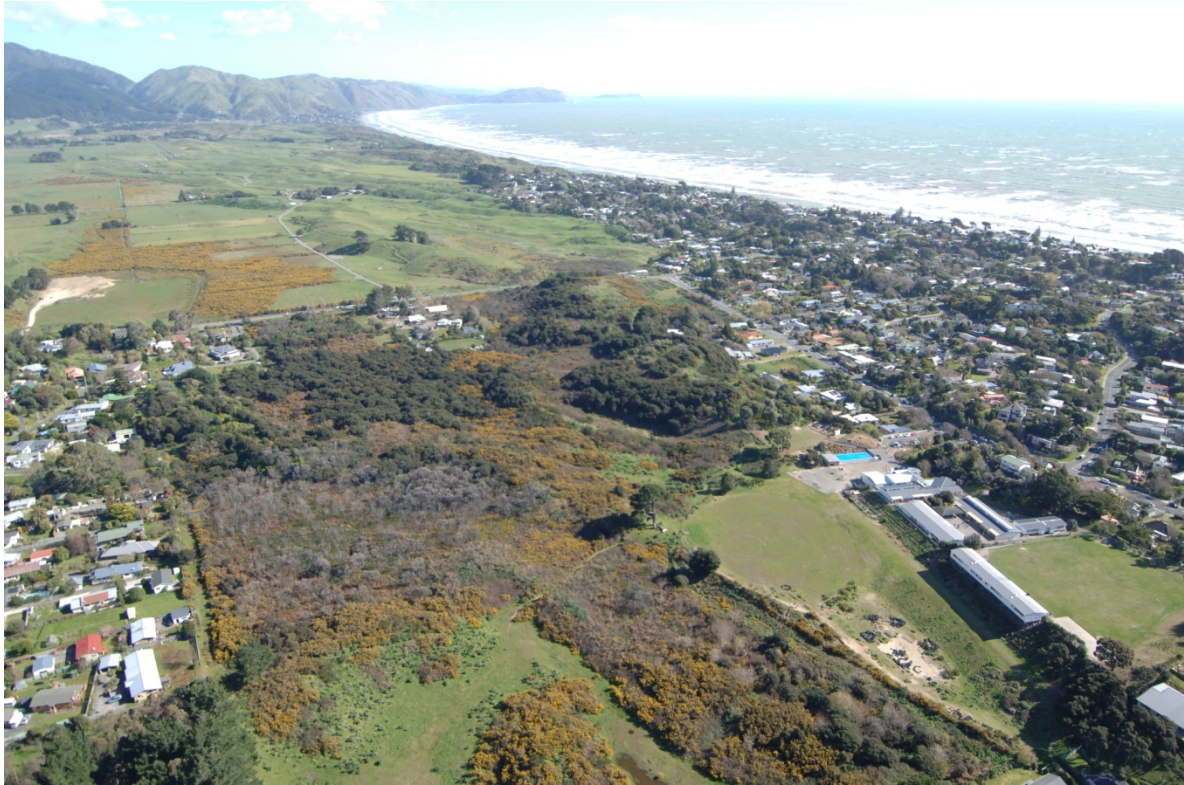
Photo 6.2: Sector 1 (Facing South)
