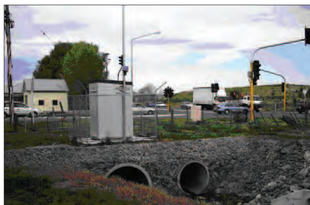
Air quality monitoring station near Meeanee Road intersection upgrade project in Napier
