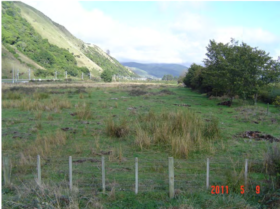
Plate One - Chainage 2500m Poplar Avenue Looking South Over Pre Load Area
