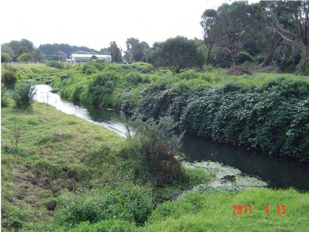
Plate Six - Waimeha Stream – protected with Super Silt Fence
