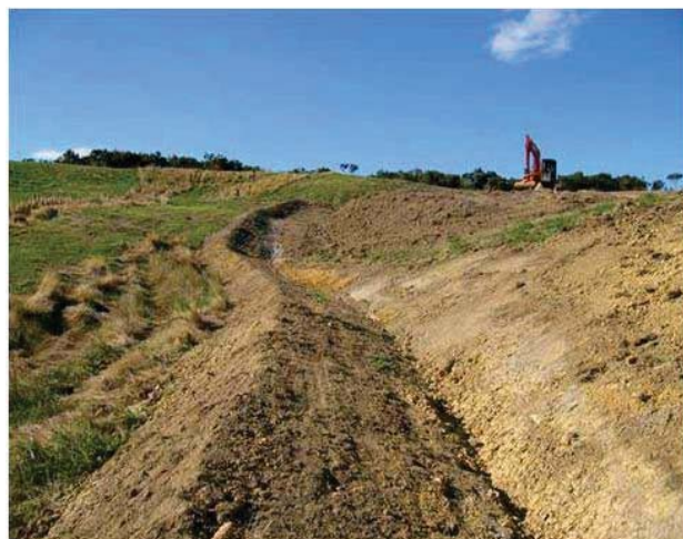
Diversion separating the clean water from the dirty water
