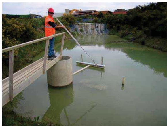
Undertaking Maintenance of a Sediment Retention Pond
