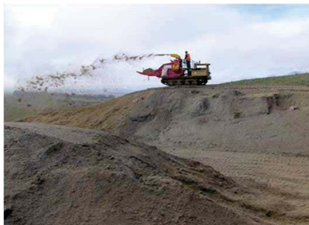
Erosion Control – Mulching
