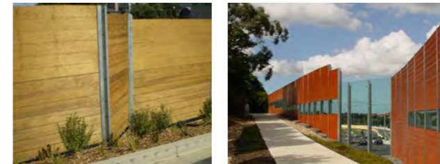
TYPE A: Timber or panelled type fence on residential boundary - can be planted with climbers or against with trees and shrubs. The fences can be offset to break up long lengths of wall. Clear panels can also be inserted. Needs specific design to ensure noise attenuating qualities.
