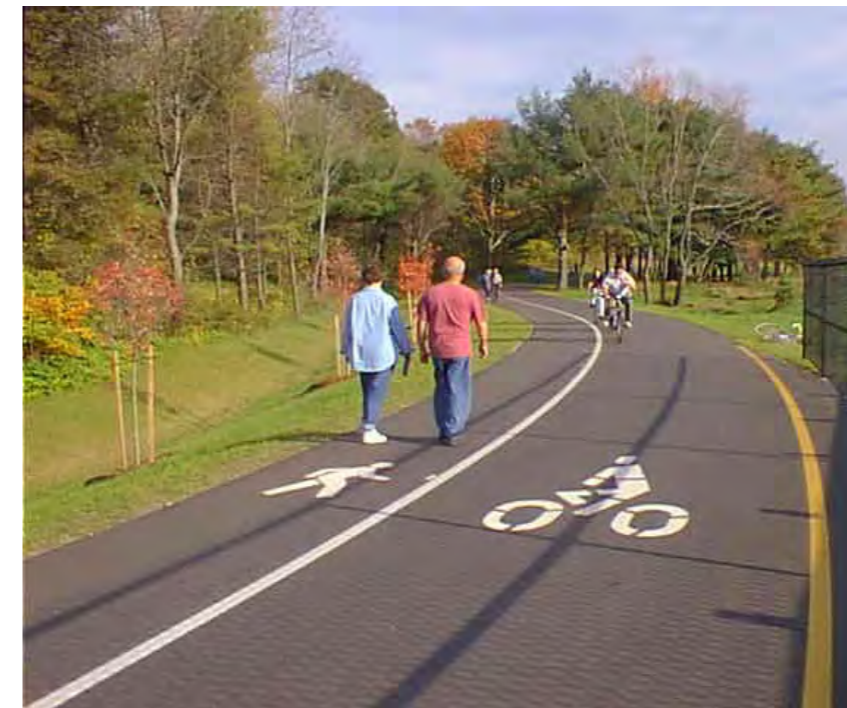
Figure 109 Indicative image of type of proposed shared cycle and walking path - shown as approximately 1m wide pedestrian and 2m wide cycle lanes
