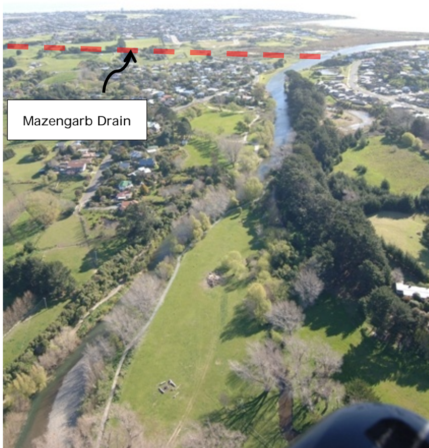
Photo 25: Waikanae River downstream of the proposed Expressway crossing.
