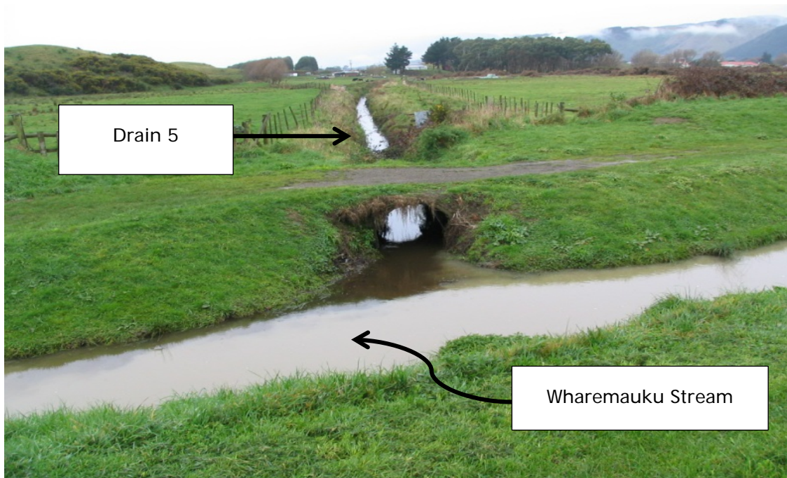
Photo 13: Drain 5- Wharemauku Stream confluence.
