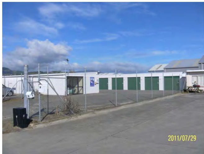
Figure 16: 17 Sheffield St – street view
