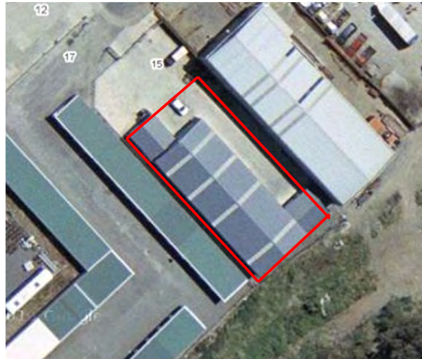
Figure 13: 15 Sheffield St – satellite view
