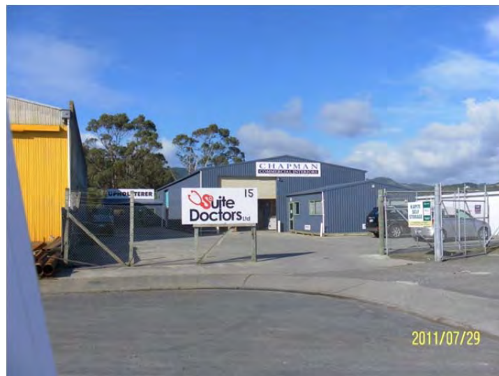
Figure 14: 15 Sheffield St – street view
