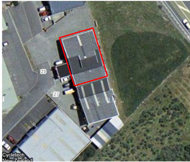
Figure 21: 23 Milne Drive – satellite view
