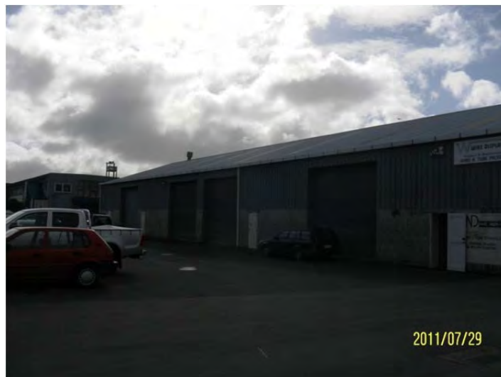
Figure 28: 106B Kapiti Rd – street view
