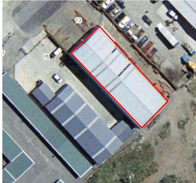
Figure 11: 13 Sheffield St – satellite view
