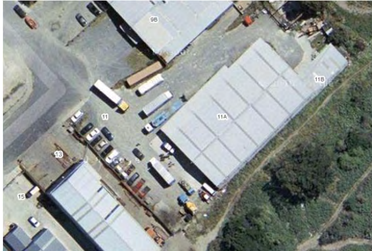
Figure 9: 11 Sheffield St – satellite view
