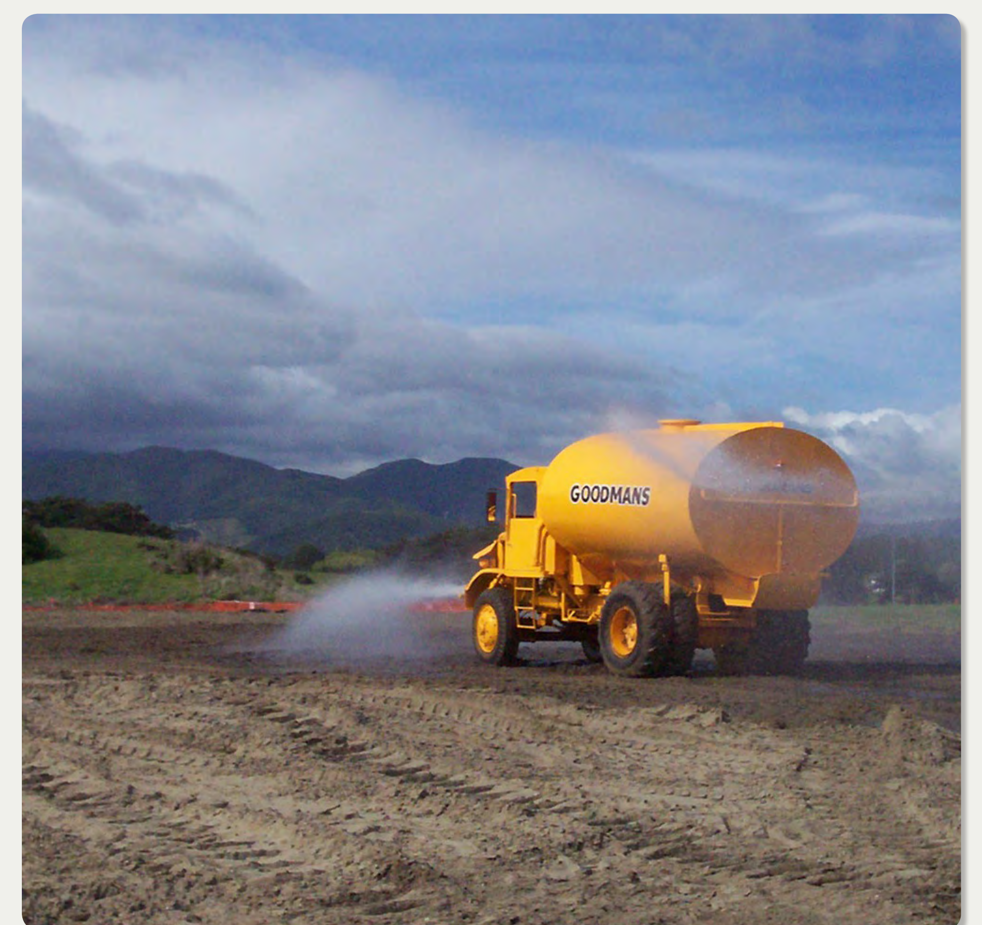
Managing dust by water dampening.
