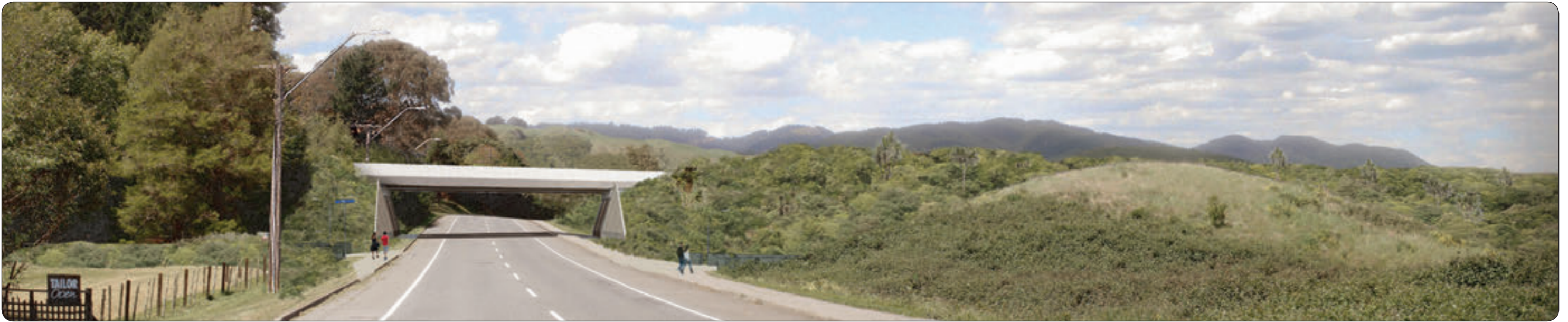
PROPOSED VISUALISATION - MAZENGARB ROAD BRIDGE (NORTH WEST SIDE OF MAZENGARB LOOKING SOUTH EAST)
