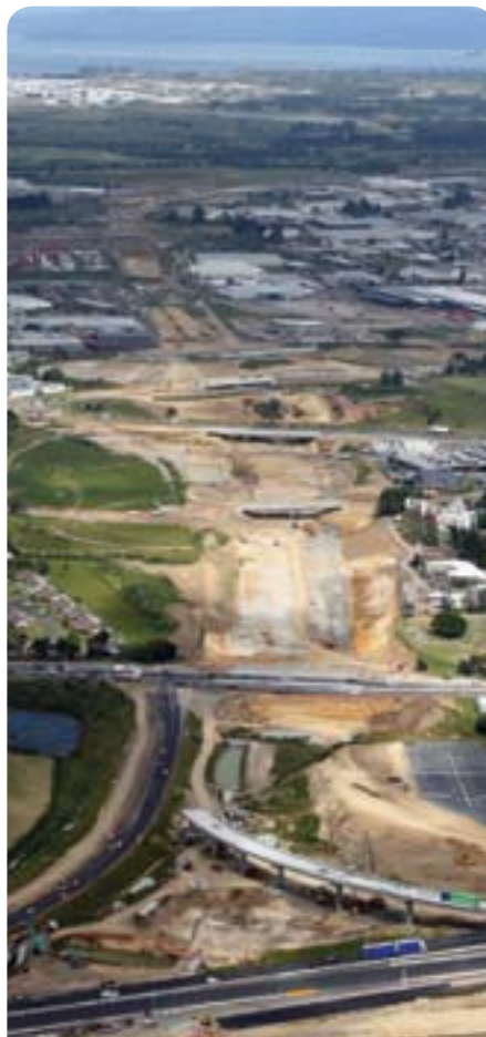
View of the motorway route looking west towards Manukau Harbour.
