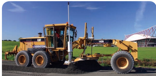
Pavement construction by the Pacific Events Centre.
