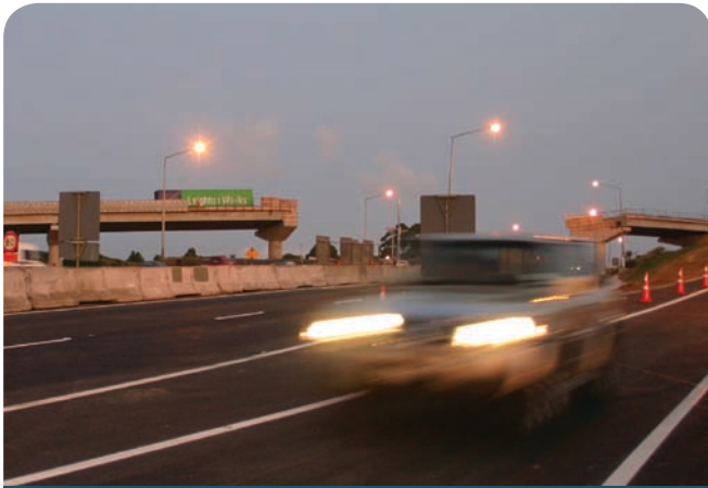
Beams will soon be installed for the SH1-SH20 Flyover.
