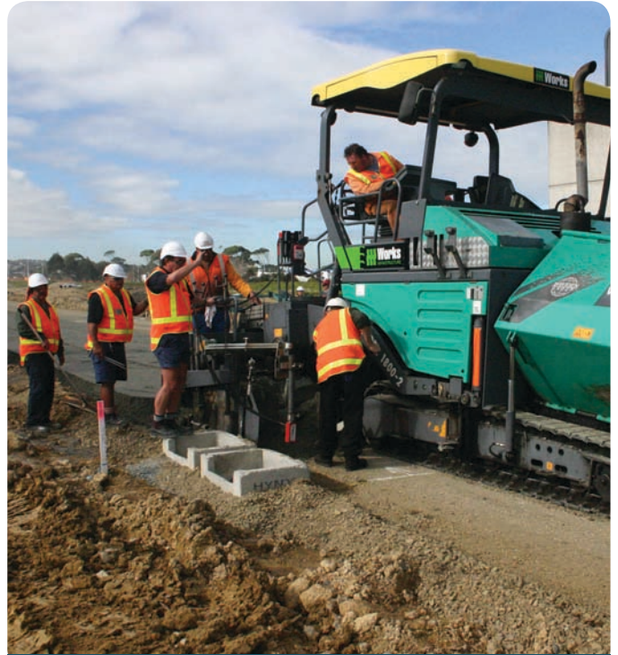
Road construction along the motorway alignment has begun.
