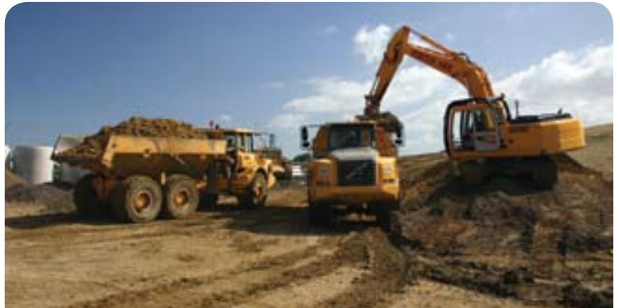
The team will be completing earthworks by the end of 2009.
