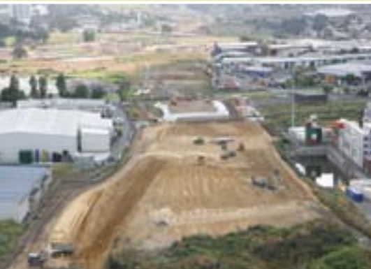
Careful steps have to be taken to manage earthworks.
