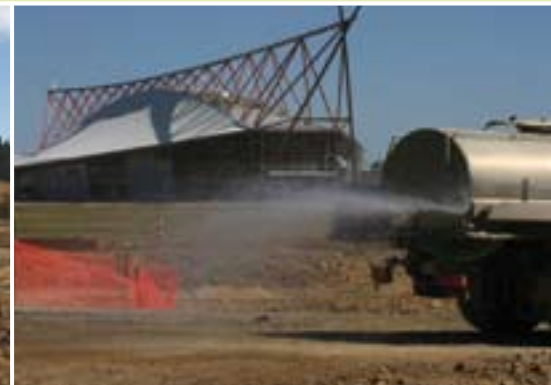
Dust is controlled by dampening down the haul roads.
