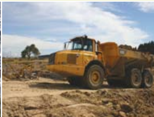
Vehicle speeds are kept low to minimise dust.
