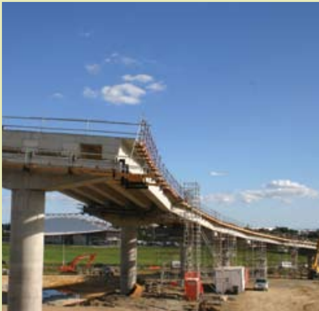
SH1-SH20 Link Flyover.
