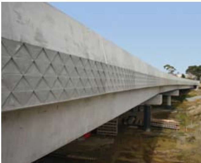
Inlaid patterns on bridge barriers reflect Manukau's Pasifika identity.
