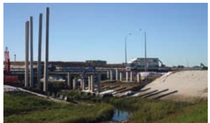
Roscommon Road is being widened for a temporary deviation.
