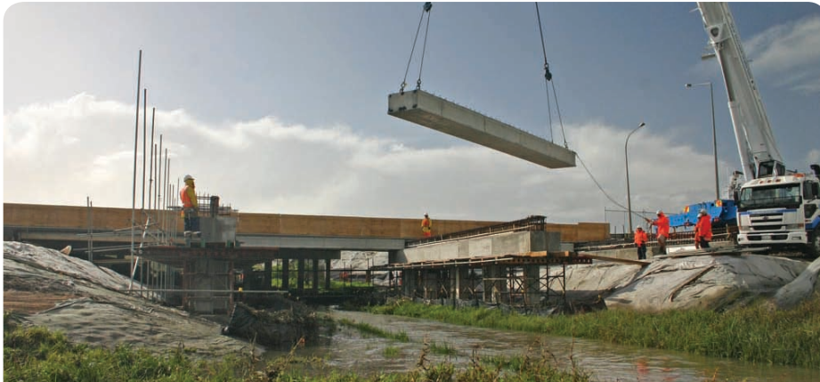
Working in close proximity to the stream requires careful environmental management.
