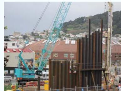
Steel sheet pile wall: the section at left has been partially inserted by a crane using a vibrating hammer; the section at right is held in place by the A-frame guide ready for partial insertion. A second crane will drive the piles down to ground level, also using a vibrating hammer.
