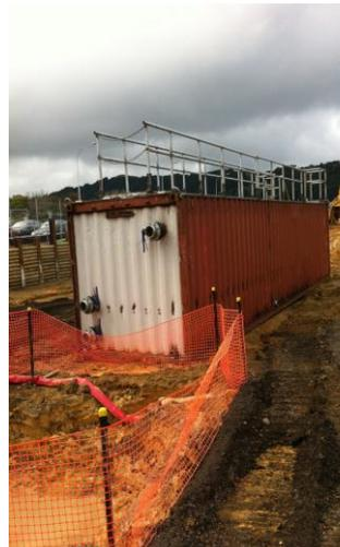
A three-stage filtration box (left) is now on site to clean stormwater and will feed into the existing catchpit (also at left) to ensure the water running off site into the city's stormwater drains will not pollute the harbour.
