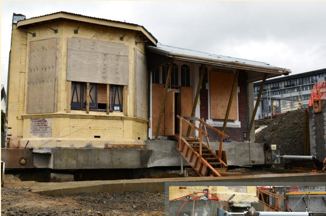
Above: The strengthened crèche ready to move. Right: One of the hydraulic rams installed for the move.
