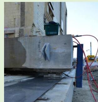
Above: Stainless steel runners laid over the concrete base are sprayed with lubricant to ease the slide. A concrete corset holds the base of the crèche tight. The hydraulic rams, in effect, pull the corset, not the house.
