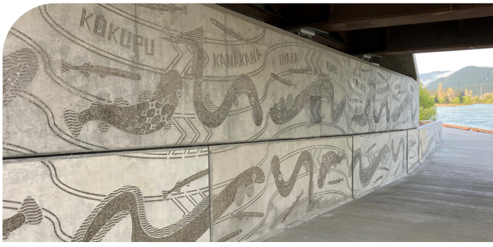
Distinctive iwi artwork on the eastern bridge abutment retaining walls.
